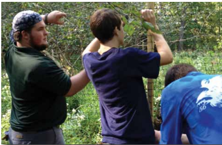
Bryce Dupes (left) works to install deer fencing at Miller Preserve.
