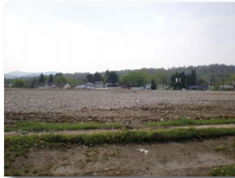
The SKF Property in Altoona, Pennsylvania, is currently undergoing preparation for commercial redevelopment, following a successful Act 2 Closure.
