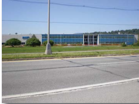
SKF Property in Altoona, Pennsylvania, before remedial activities.
