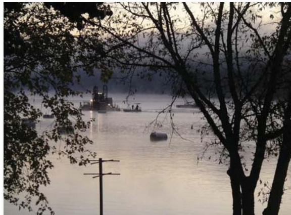
Dredging activity on the Emory River.
