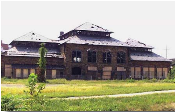
Foundry Building Before Renovation
